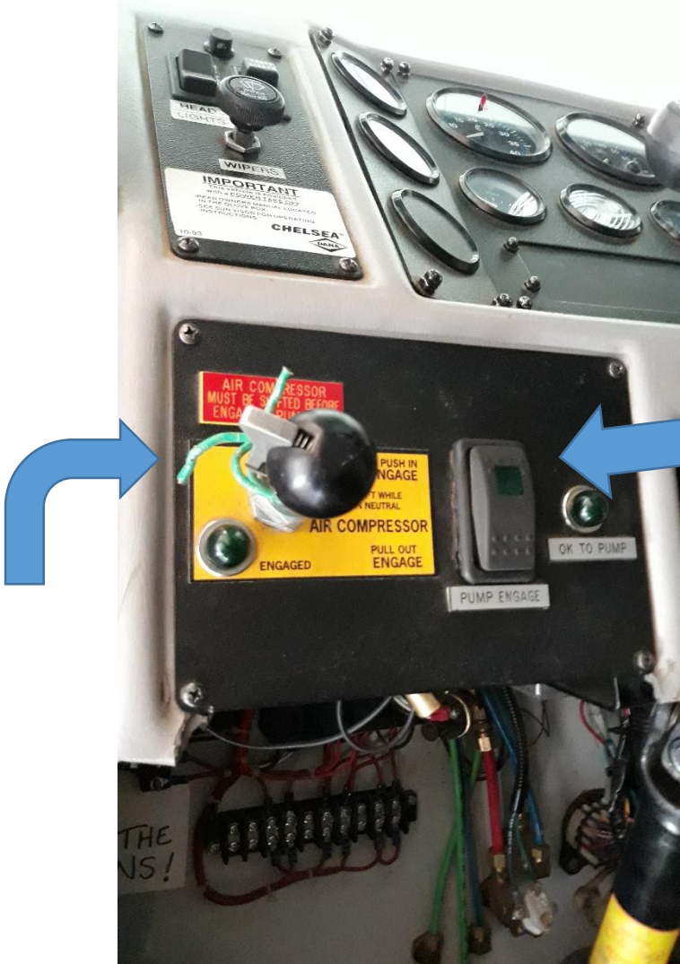
Compressor control switch
